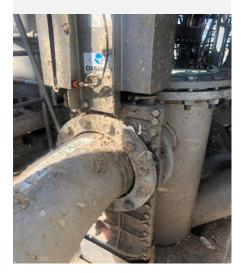
The Spanish Packaging Corrugated Cardboard Paper Mill discovered their Pulping System was producing a larger reject concentration than expected. This larger concentration rejects were causing clogging situations in the HDC valves and were resulting in reduced valve live
